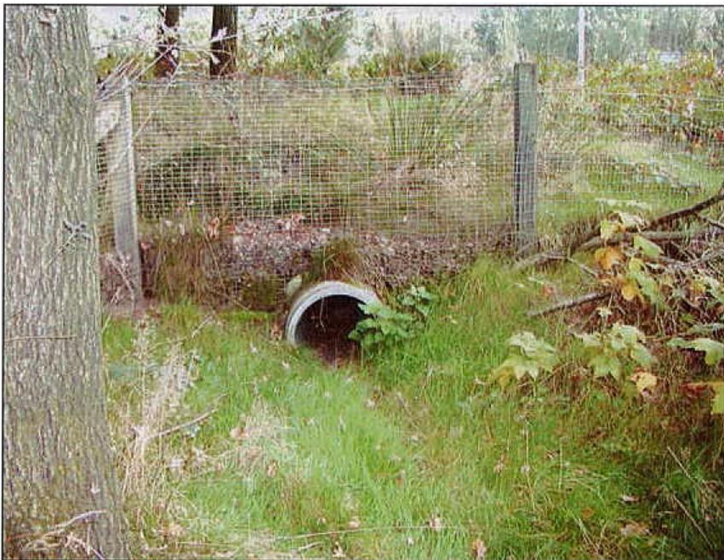
Figure 11. Another example of a badger crossing from The Netherlands. Note that fencing is only 3 feet high. This structure and fencing also work well for other small mammals and amphibians.
