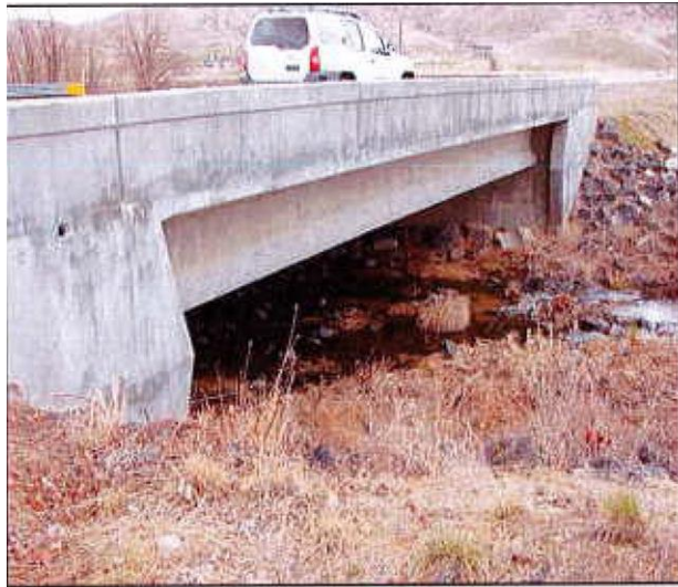
Figure 1. Dry Creek Bridge.
