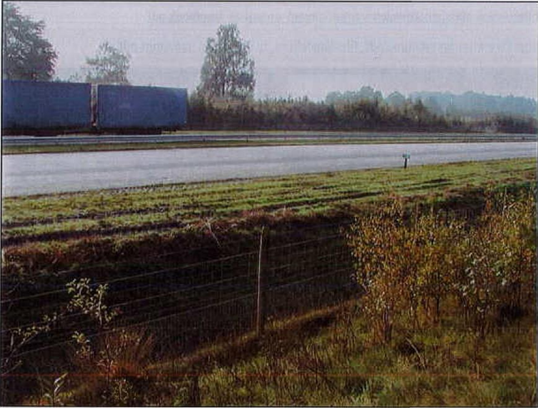
Figure 19. Screening is used on the bottom half of this wildlife fence in The Netherlands to prevent amphibians and small mammals from crossing onto the highway surface.
