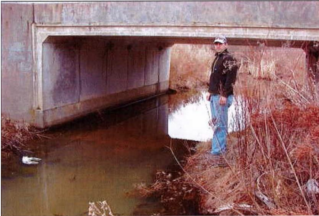
Figure 7. Bridge at crossing of South Fork of Willow Creek. Bridge provides good fish passage, but limited passage for terrestrial species. Kenn Hardin from Environmental Conservation Services in photo.
