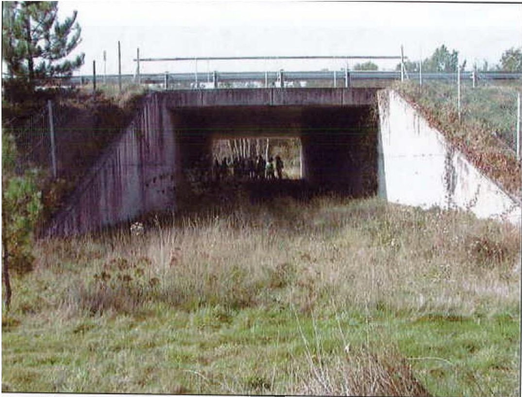
Figure 14. Large box culvert wildlife underpass in France.
