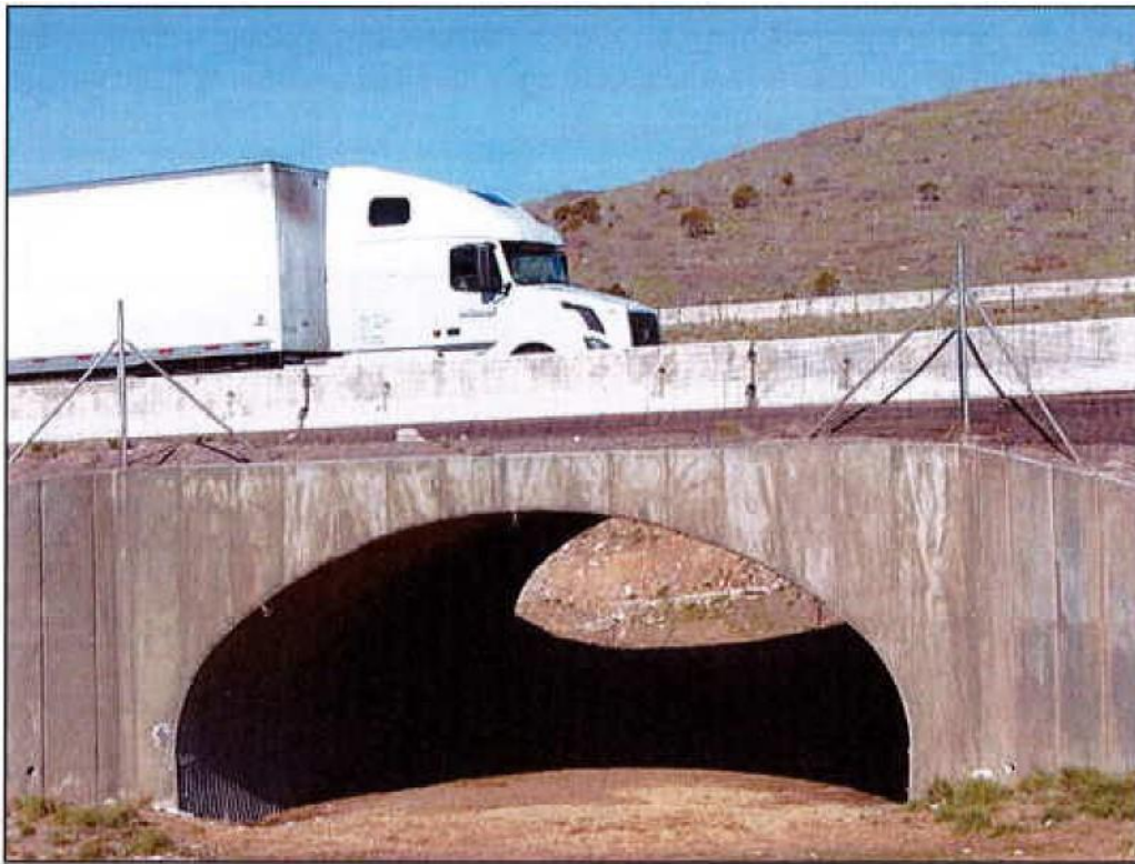
Figure 13. Steel arch wildlife crossing on 1-15, Utah.
