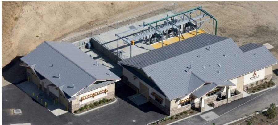
Figure 5-1 Avimor Water Reclamation Facility
